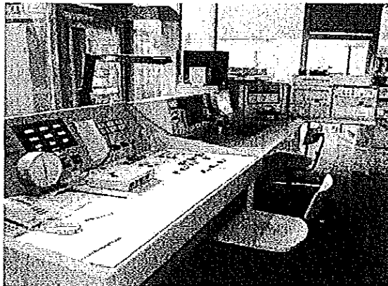
Control station for tests up to 10kA
